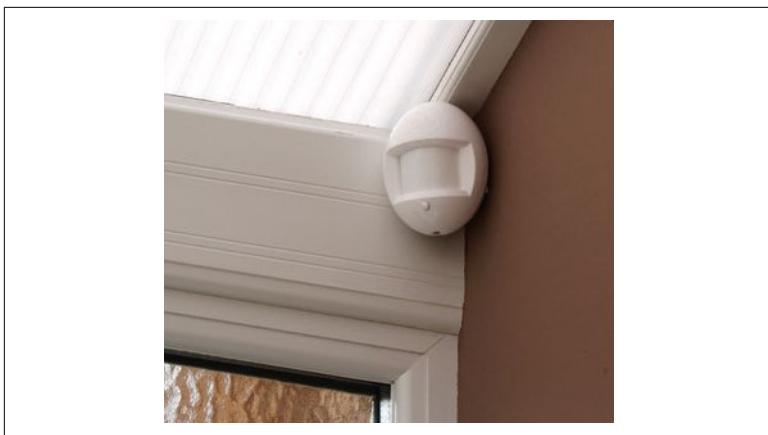
Figure 1-18. A typical presence sensor, hidden in the corner of a room
